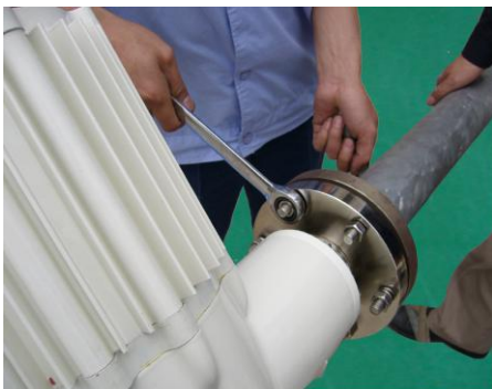
5、 ATTACHED THE FLANGE AND TOWER WITH LOCKNUTS
