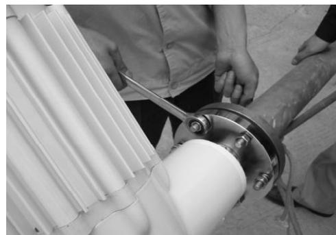
(8) Mounting flange and tower with locknuts.
